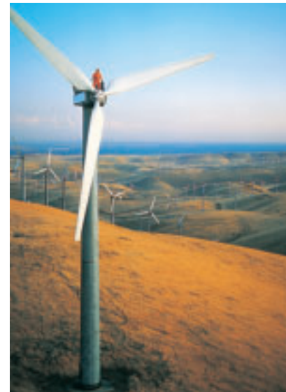
Figure 25 Windmills work on the same basic principles as a power plant. Instead of steam turning a turbine, wind turns the rotors. Describe some of the advantages and disadvantages of using windmills.
